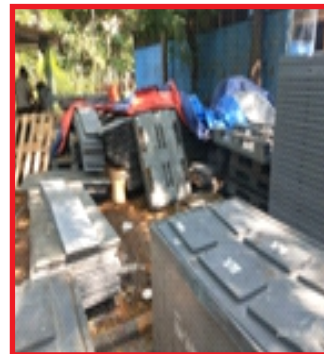
Packing materials are lying in the open area
